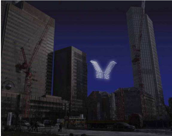
Caption 2: Although not yet completed, the TaunusTurm office building is already a work of art. For the Luminale, artist Laura Bernadet has delineated the future tower block head with white lines of light.
