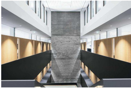
Caption 4: Using this lighting solution largely based on LED and further supported by presence detectors, the i+R Group was able to cut lighting-related energy consumption by up to 70 percent.
