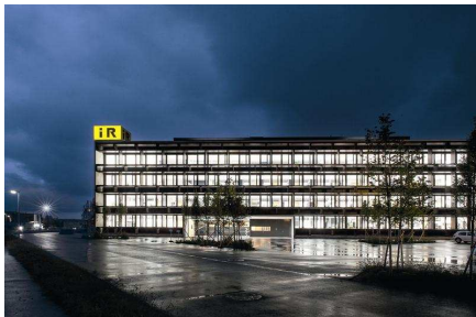
Caption 1: The i+R Group headquarters is the first LEED Platinum certified building in Germany, Austria and Switzerland.
