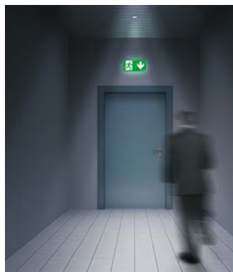
Illustration of the pictograph with a luminance level of 200 cd/m 2
