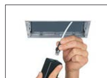
Connect luminaire to electrical power supply
