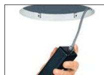
After applying plaster, connect the luminaire to electrical power supply
