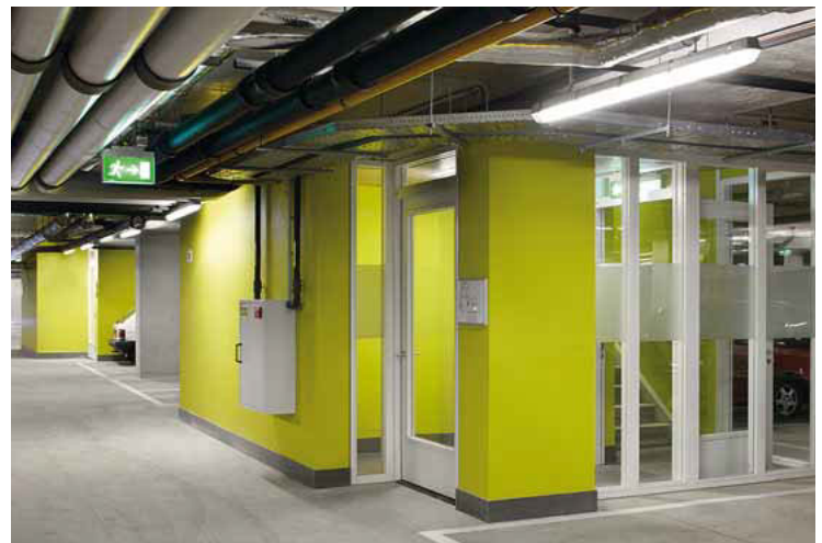
Underground car parks and plant rooms
