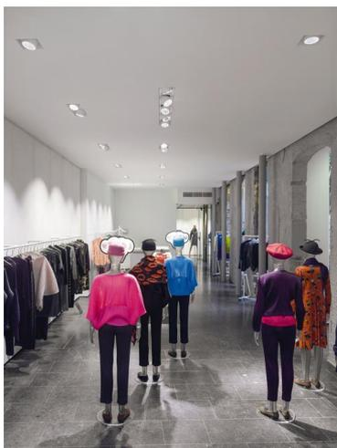
**Image 3:** Each dummy is highlighted by a pair of accent spotlights from the INTRO lighting system, which is fitted flush into the ceiling. One spotlight with a focused distribution and one with floodlight characteristics offer the optimal combination.
