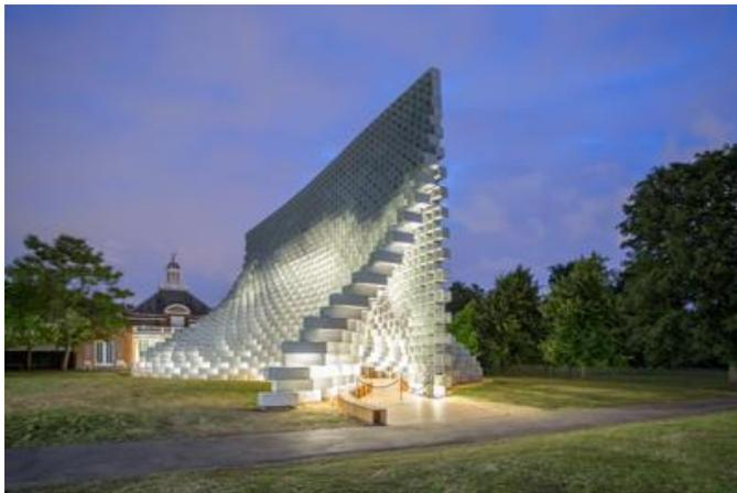
**Fig. 1:** BIG’s [Serpentine Pavilion](#) of this year 2016 takes the form of a wall created from stacked, open-ended rectangular boxes.
