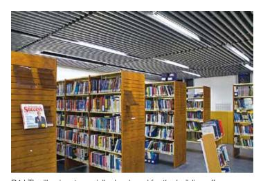
B4 I The illuminant specially developed for the building offers a very high efficiency despite its very small dimensions and fulfilment of the anti-glare specifications. The illuminant used is a visible, innovative T5 lamp.
