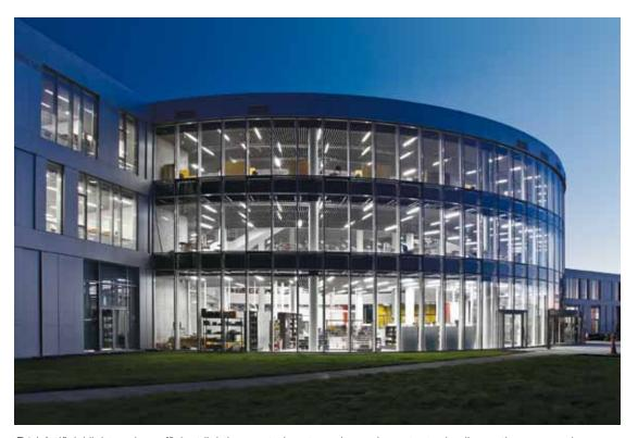
B1 I Artificial light and an efficient lighting control system play an important role all over the campus because of the typical lighting conditions in northern latitudes. The individual departments are arranged around the central circular hub in the shape of a star.
