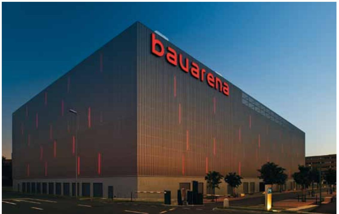
B2 | Via an intelligent DMX control system, Zumtobel's Hilio LED light lines have been matched perfectly to the red Bauarena logo, in terms of colour. The sophisticated lighting concept therefore not only catches people's attention but also creates a distinctive design outside and inside the building.
