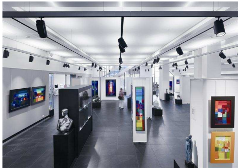
Picture 2: In order to set the perfect lighting stage for presenting the artworks, a total of 230 spotlights were installed on Supersystem tracks.
