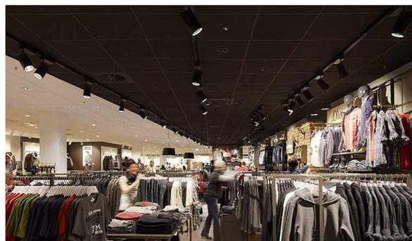
young fashion accessories, appealingly and to full effect. Zumtobel used its latest Lyon LED spotlight range and its Cardan LED lighting system to satisfy this requirement. The Lyon spotlight's sophisticated design accommodates a unique lens/reflector system that allows for high-precision, homogeneous accent lighting with a variety of beam patterns. With a stable warm white colour temperature of 3000 K and excellent colour rendering ( $R_a > 90$ ), the LED
