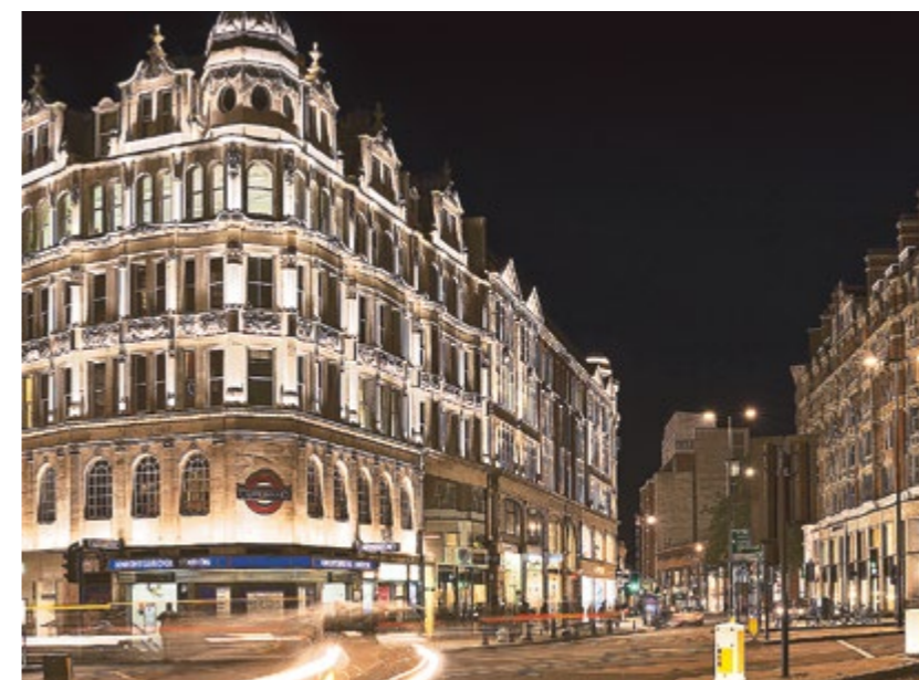
Facade of the Knightsbridge Estate, UK
