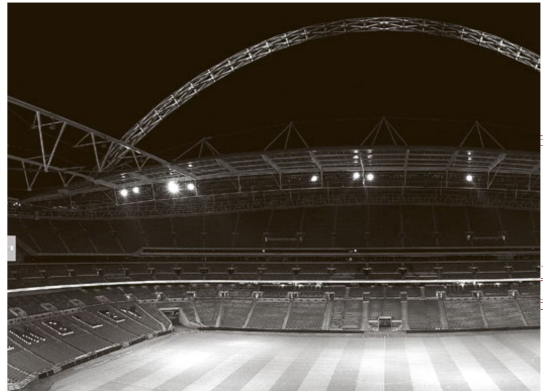
Lighting for indoor and outdoor sports Wembley Stadium connected by EE, UK
