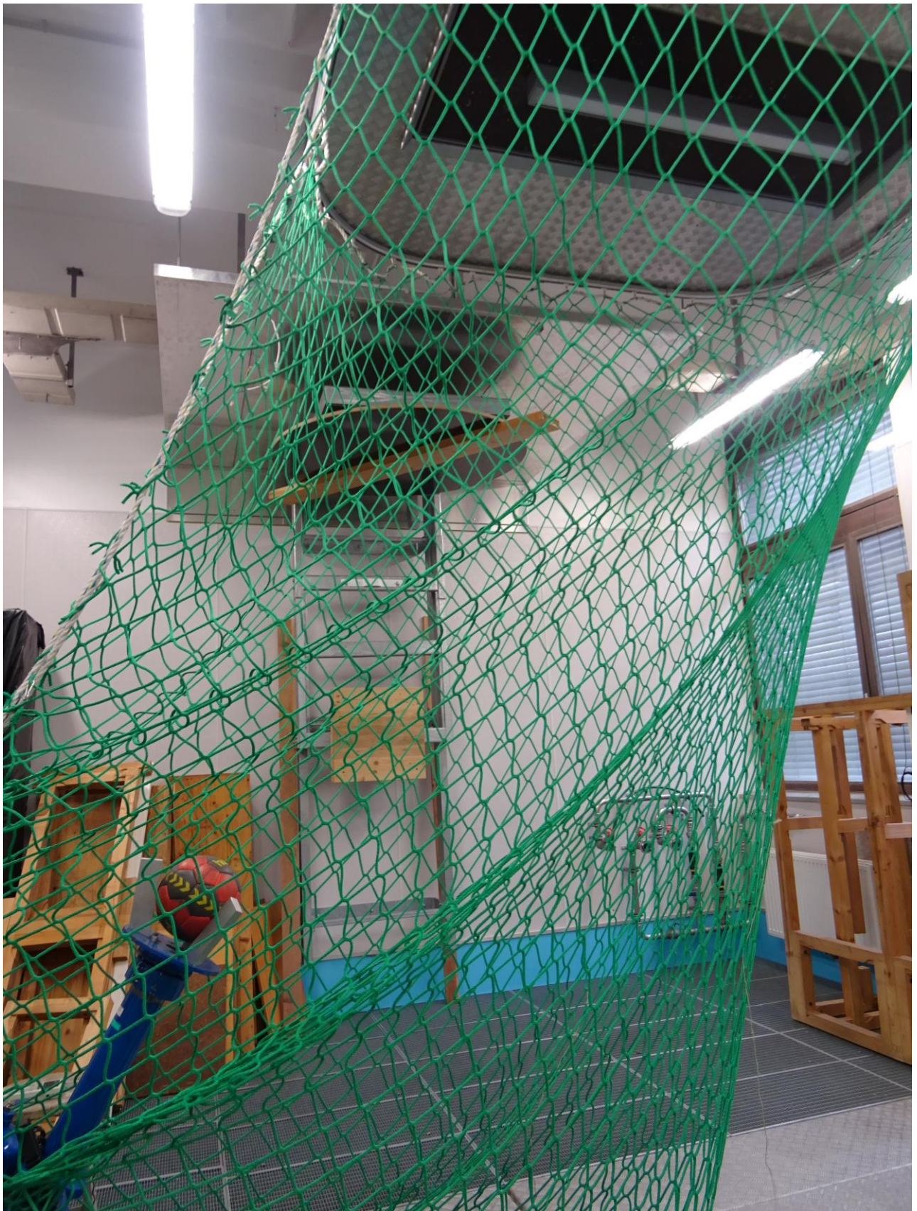
Figure 12: SLN2-B 1600-840 L1250 PC/PCO/DD LDE + SLN2 C MSC L 1250 SR – direct mounting on ceiling
