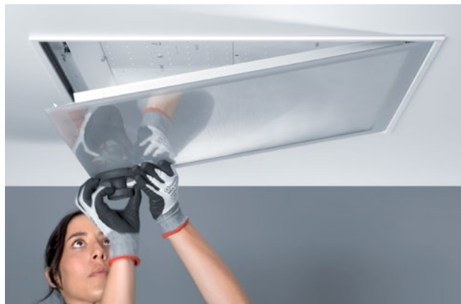
The CLEAN II supreme essential offers easy maintenance and installation without removing the Light Engine and is designed to be future-proof.
