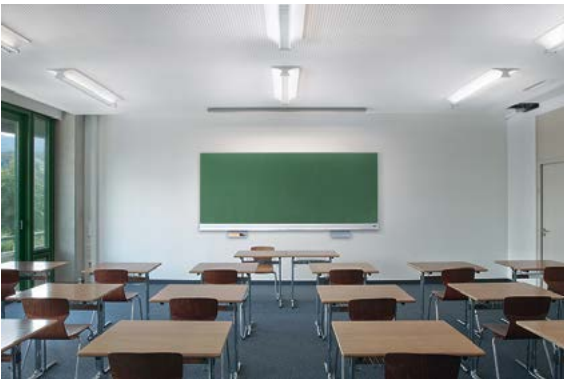
Lighting concept for classrooms
