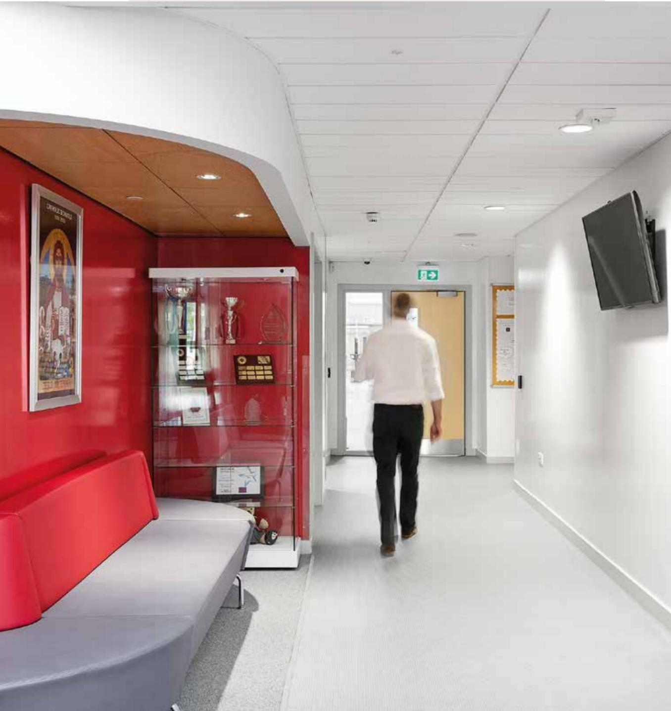
SLOTLIGHT has provided a truly integrated, low energy solution for the project with excellent colour rendering of  $Ra > 80$ , lighting efficiency of up to 92 lm/W and a service life of 50,000 hours.
