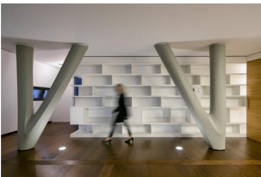
Photo 5: Round PASO II LED fittings have been recessed into the floor to provide efficient general lighting.
