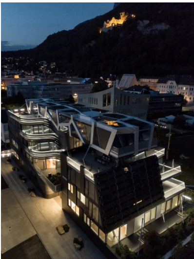
Photo 6: With its futuristic elegance, green values and experimental planning process, the Active Energy Building in Vaduz is a real flagship project for energy-efficient architecture.
