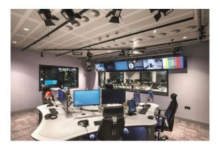
**Image 4:** Outstanding light quality and excellent colour rendering: in the broadcasting studio, Zumtobel uses a powerful combination of spotlights, including SUPERSYSTEM and PANOS evolution downlights.
