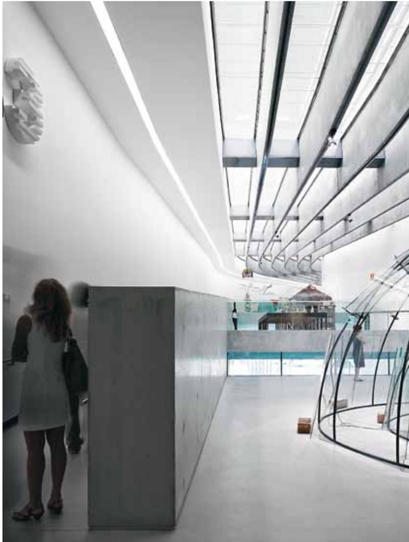
B6 I All the technical elements are accommodated in the complex luminous ceilings. The general illumination is provided by light bands with dimmable fluorescent lamps fitted behind light-scattering translucent acrylic glass. Spots offer additional point illumination.
