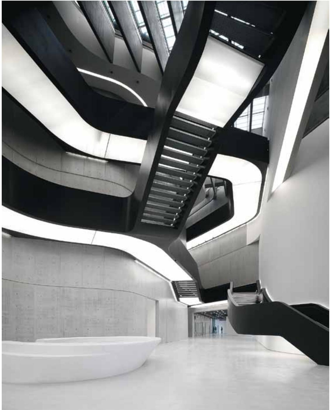
B2 | The soft light not only radiates downwards, but also diffuses upwards through the grating of the steps and pathways. Light bands hidden in the handrails follow the stairs as a source of indirect illumination.
