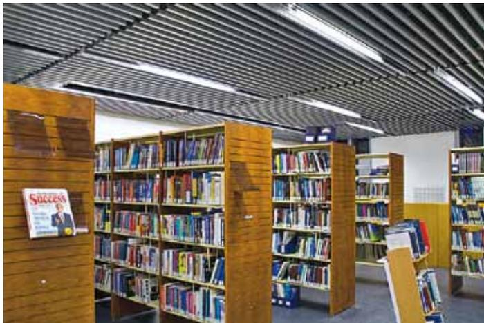
B4 | The illuminant specially developed for the building offers a very high efficiency despite its very small dimensions and fulfilment of the anti-glare specifications. The illuminant used is a visible, innovative T5 lamp.
