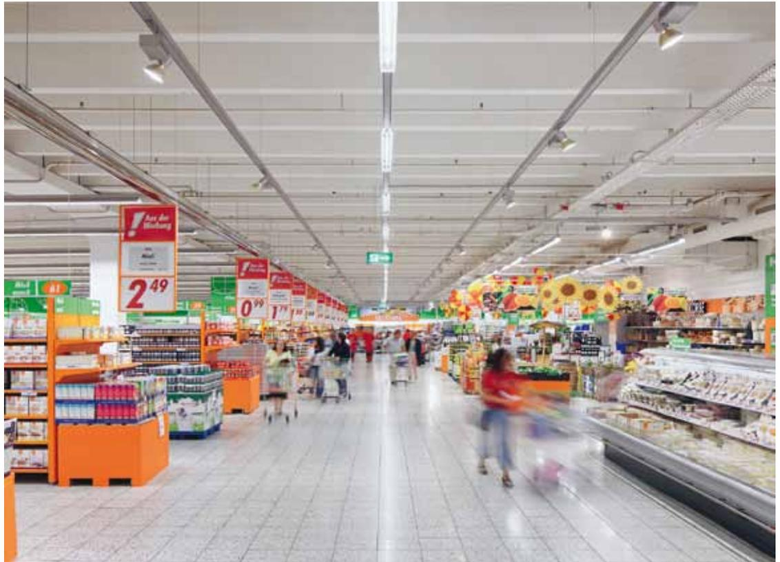
B5 | Using a variety of lighting modules, light sources and optics, the modular Tecton continuous-row lighting system can be modified as required. Owing to its high flexibility, the lighting concept can respond perfectly to varying product presentations according to seasons.
