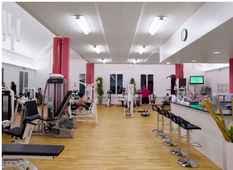
B5 | Even in the “Benefit” sports area, people work out under mellow lighting conditions: the Mellow Light IV surface-mounted luminaires chosen for this purpose create an atmosphere of well-being that is inspired by daylight.
