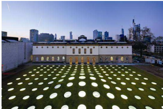
Caption 1: One hundred and ninety five circular skylights allow daylight to flood into the garden halls and transform the garden into a gleaming carpet of light at night.
