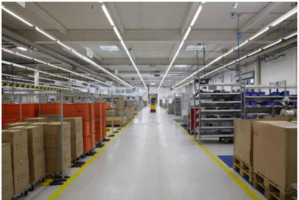
B2 | Improved lighting quality, less energy: the Tecton continuous-row lighting systems are controlled via an intelligent lighting management system. In this way, just enough artificial lighting is added to provide the optimum illuminance level of 500 lux required. The daylight-based lighting system saves up to 50% of energy.
